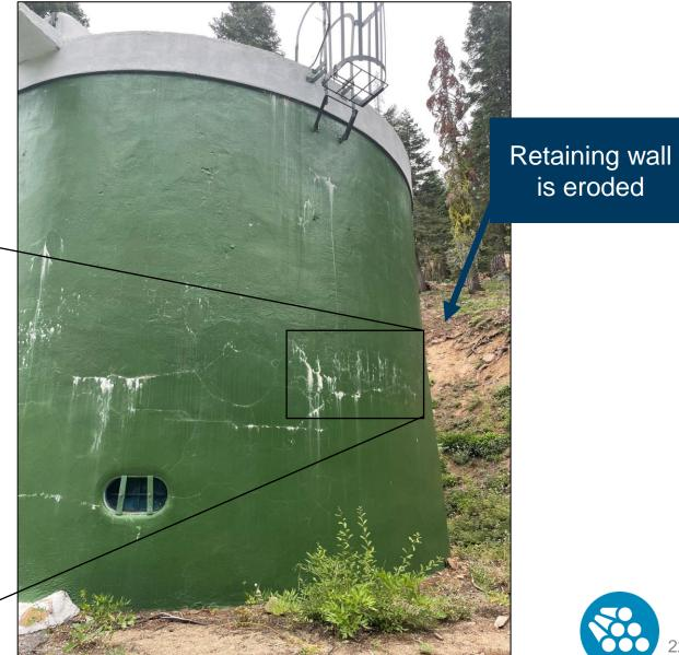
// The Alpine Meadows Estates Well #1 (AMEW #1) has hydraulic and operational issues that lead to advanced degradation and redundancy concerns
