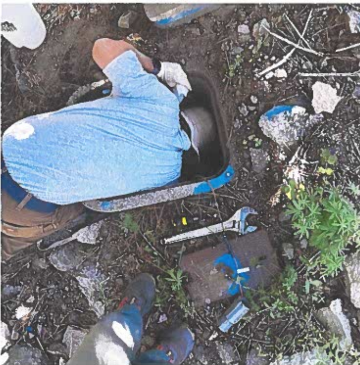
Changing Failed Water Meter
