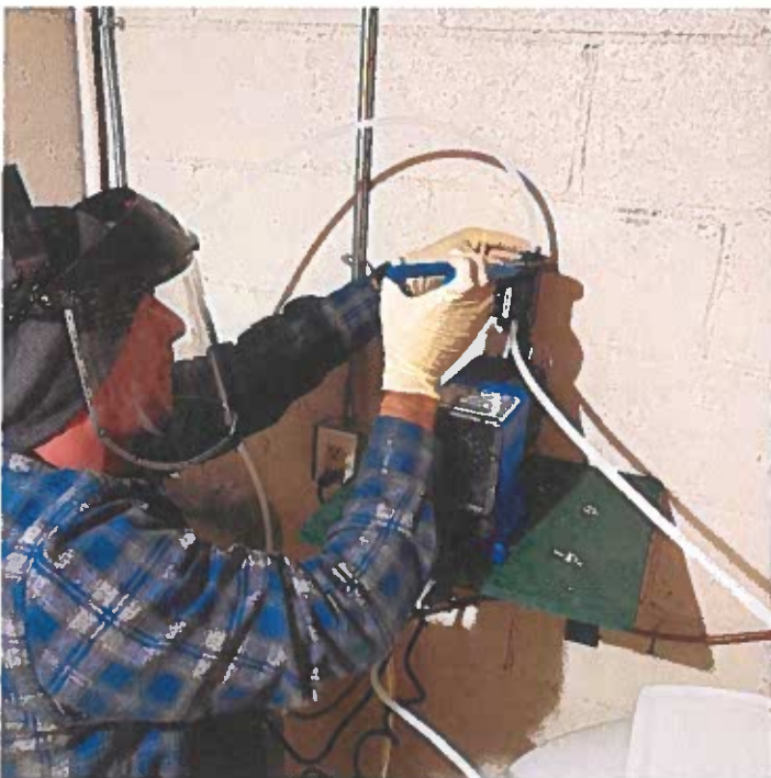
Chlorine injection pump rebuild
