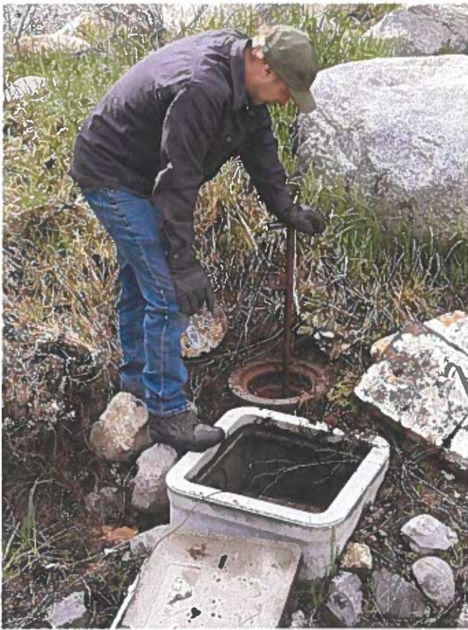
Turning on seasonal water service to the boat inspection station.
