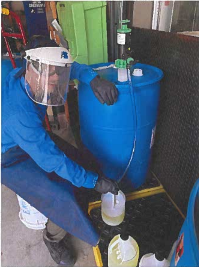
Operation of the bulk Chlorine fill station.
